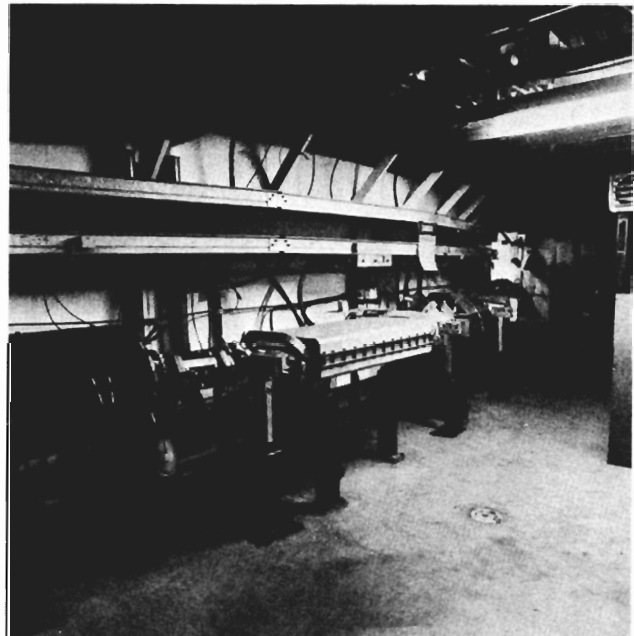
Fig. 13. Fermilab 200 MeV Storage Ring.
