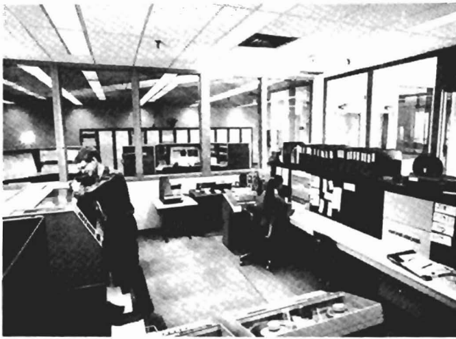
Fig. 11 Central control computer.
