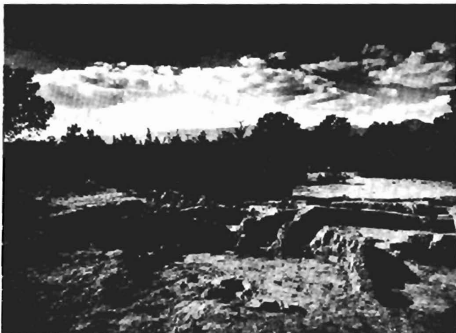
Fig. 1 LAMPF Site before construction started
