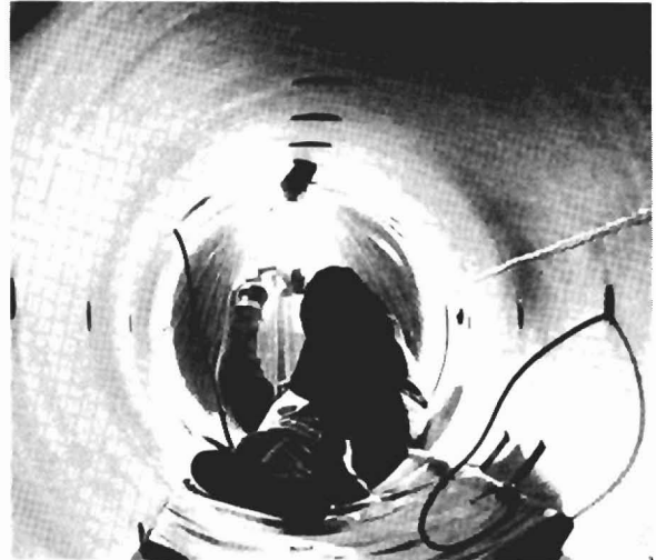
Fig. 6 Interior steel weld 201 MHz tank section joint
