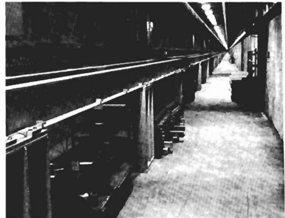
Fig. 8 805 MHz tank support structure
