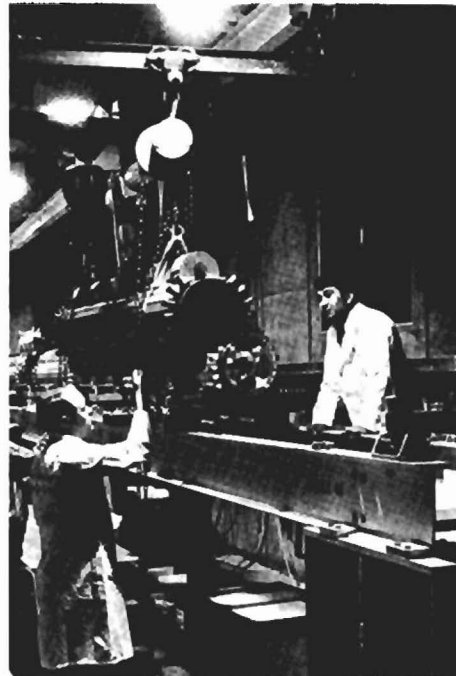
Fig. 13 805 MHz tank section hoisting into position on rails
