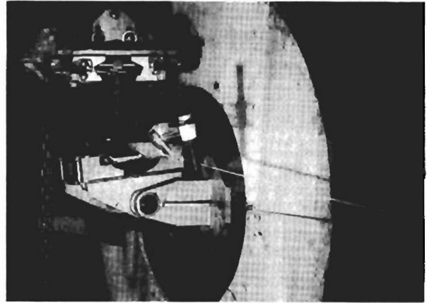
Fig. 8. Press being set up on the winding.
