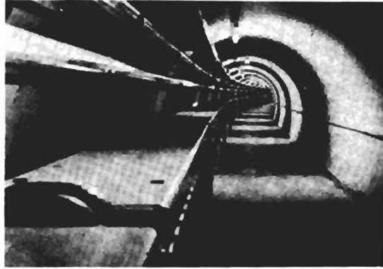
Figure 5. Main Accelerator Tunnel
