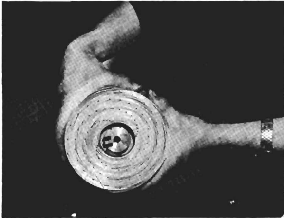
Fig.2c Tape coil fabrication.
