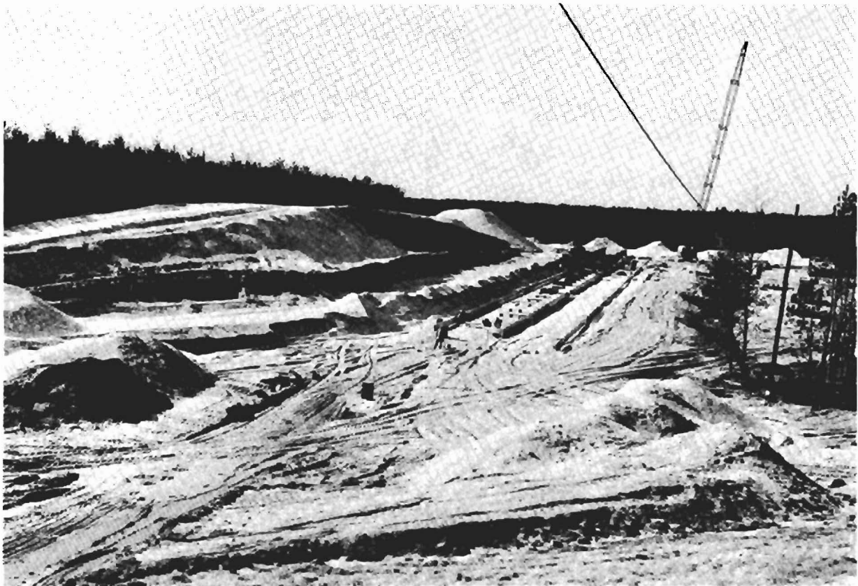
Figure 2) Linac building site development
