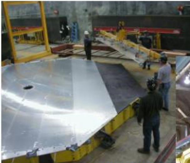
Steel Welded and modules placed.
