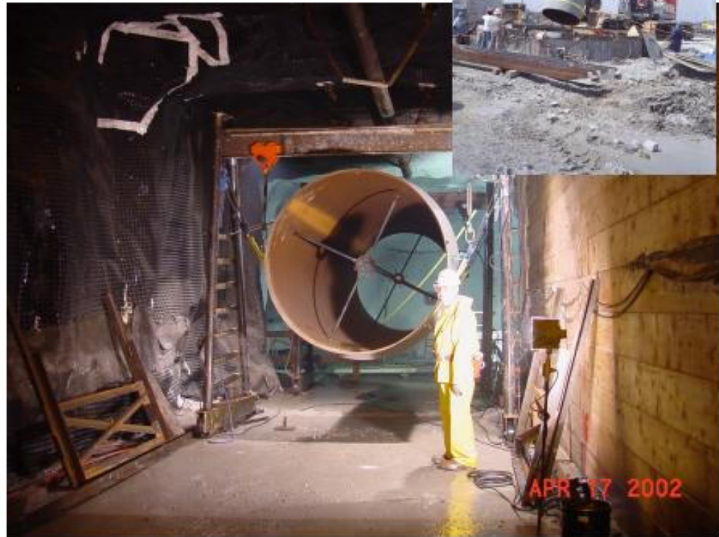
The first section of decay pipe is hoisted into place.
