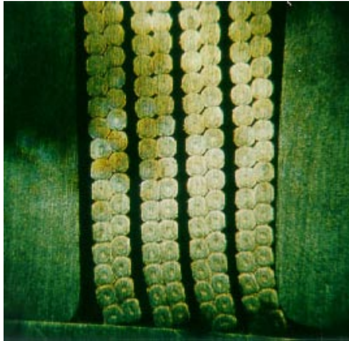
Figure 8: Close up view of the bottom surface of conductor group 1.
