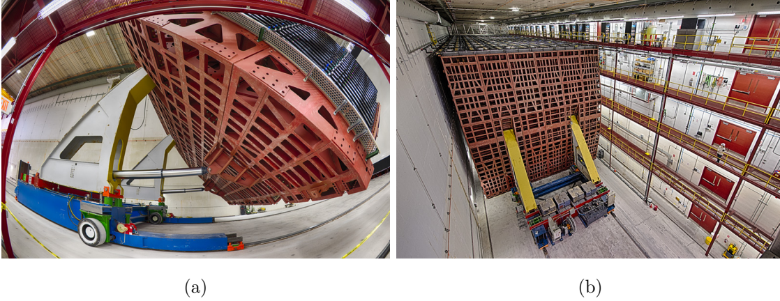
Figure 3.11: Photographs of the FD hall. The detector was assembled in 1 kilo-tonne blocks of planes horizontally, before being lifted and pivoted by 90^\circ into position ( left ). The complete detector is shown on the right [55].
