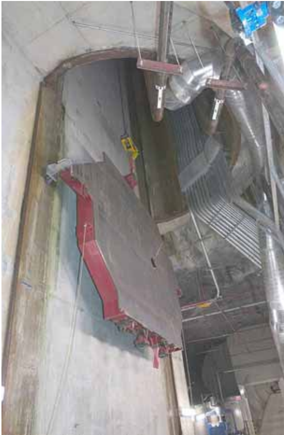
Fig. 9.2: View from the bottom of the MINOS shaft as a MINOS near detector plane comes down the shaft. The D-shaped shaft cross section is evident. The MINOS module shown is \sim 4.5 m wide by \sim 3.5 m high by \sim 0.2 m thick (including the red strong-back frame).
