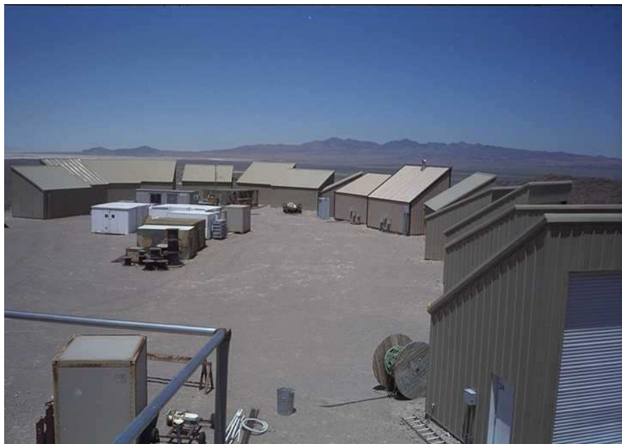
Figure 3.1: Overview of the HiRes-2 site on Camel's Back Ridge. The 21 mirror buildings are arranged in a circle around a central facility.
