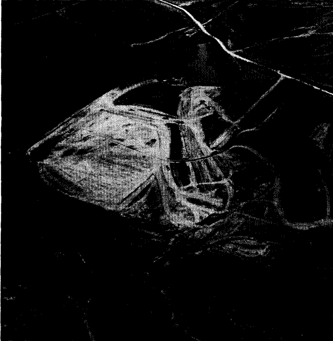
FIG. 9-1. Aerial photograph of the ongoing site-clearing and grading activity at the IR5 site.
