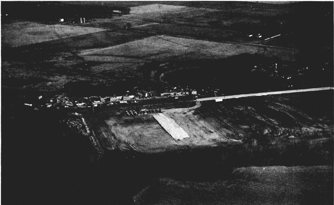
Fig. 1. A recent aerial photograph of the construction site, looking south-east. The linac building is behind the parking lot. The booster-enclosure excavation is to the right. The small white dots to the left and right of the far side of the booster excavation are main-ring survey monuments.
