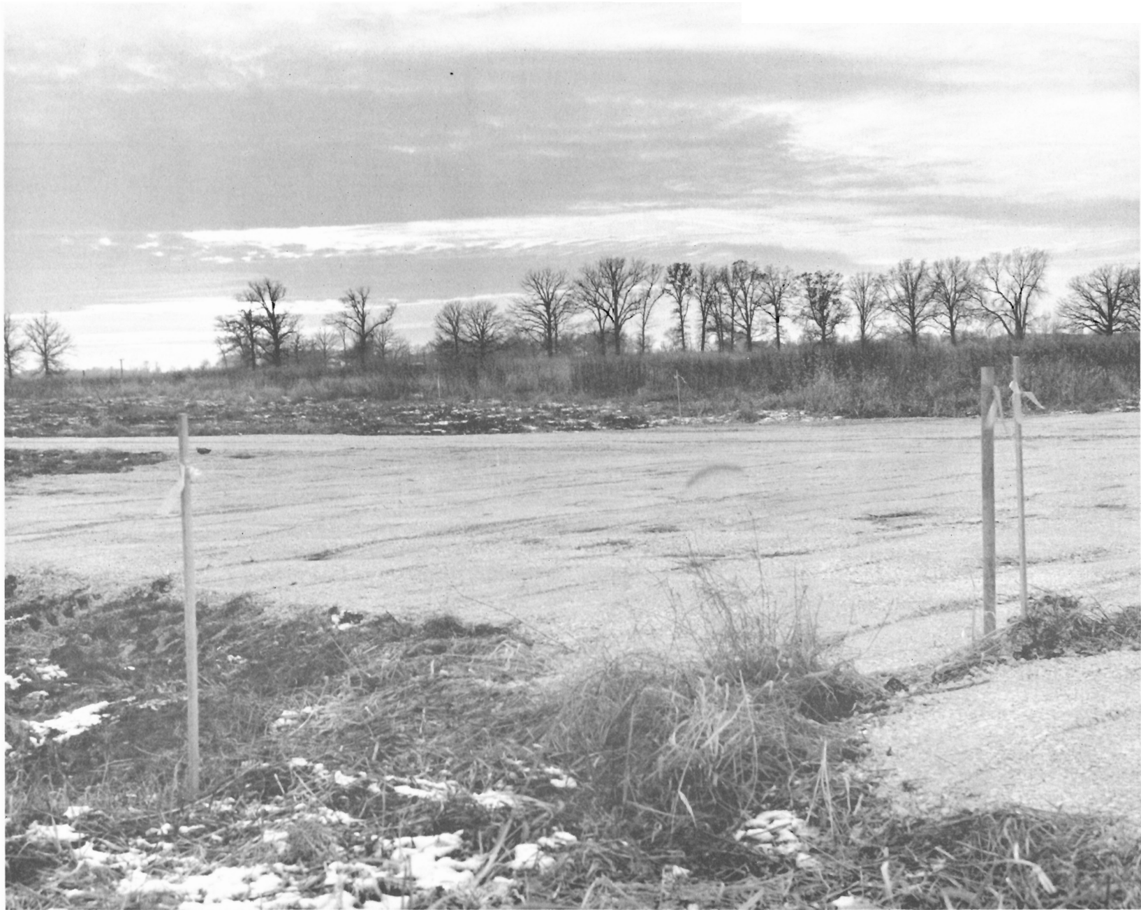
Fig. 2. Site of the Groundbreaking, looking across the temporary parking lot toward the site of the Linac Enclosure.
