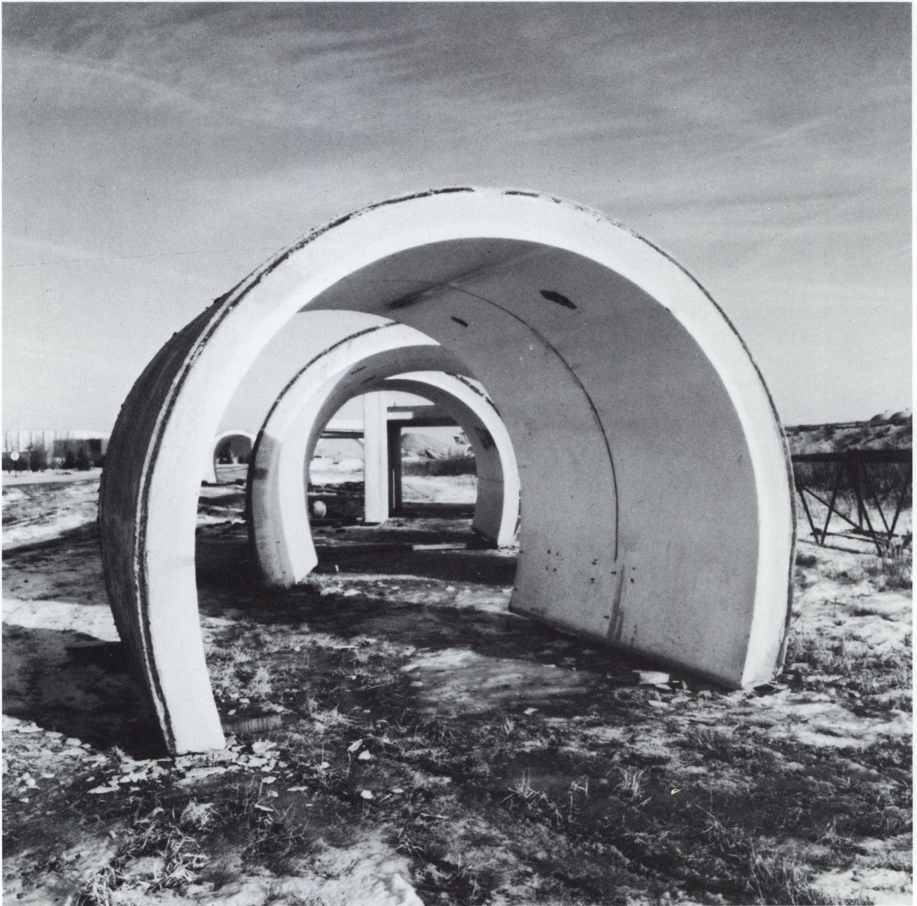
Original Main Ring tunnel sections, buried in 1970-71, replaced this year with larger sections to accommodate the B0 overpass currently under construction.
