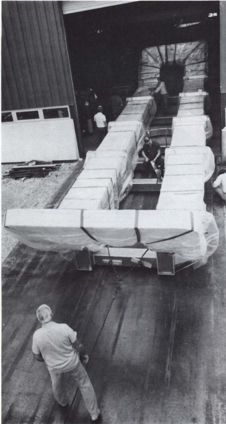
Riggers move the four-layer coil out of Industrial Building 4 on its way to the Meson Detector Building.
