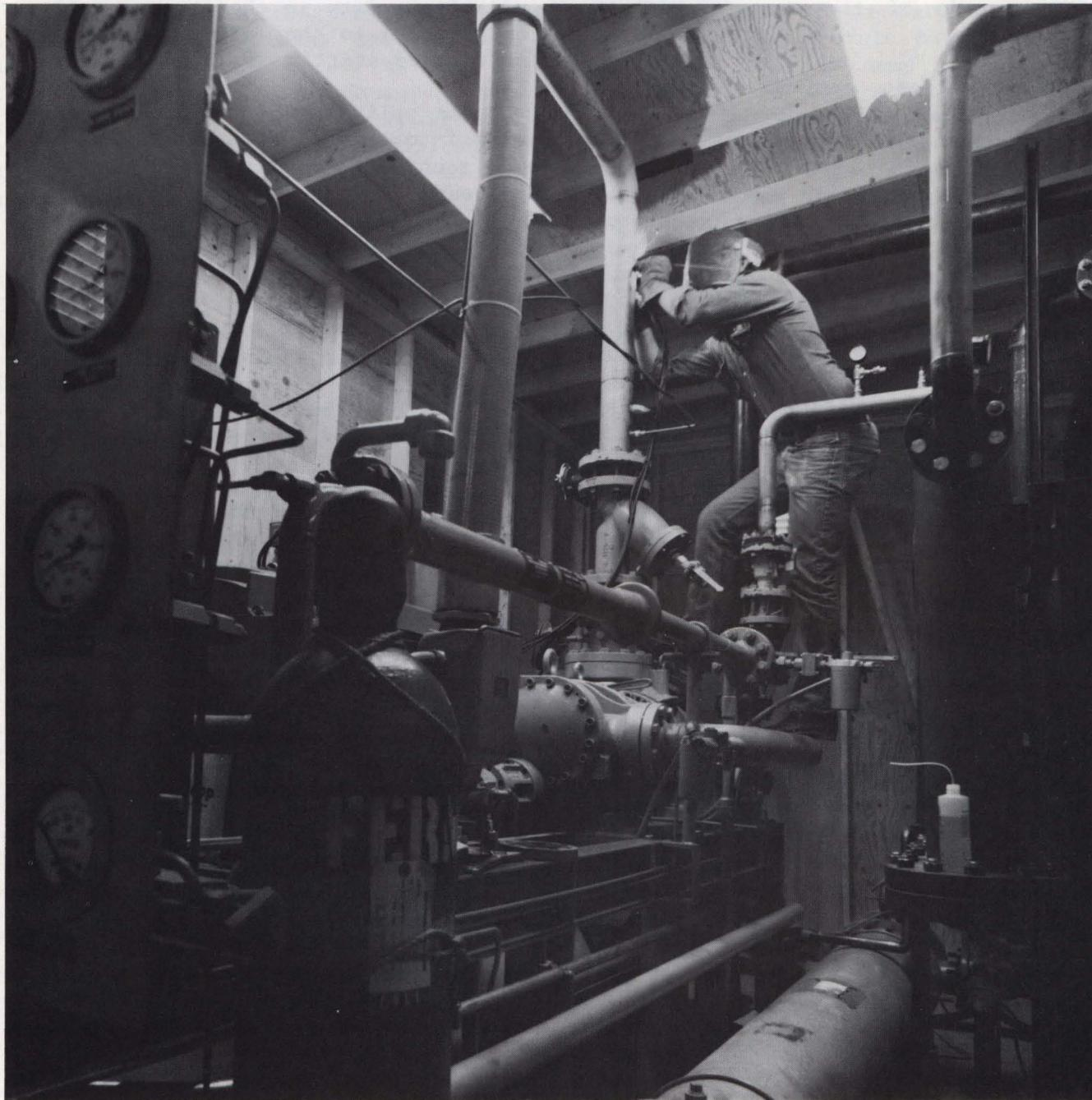
A welder works on superconducting refrigeration-system installation.
