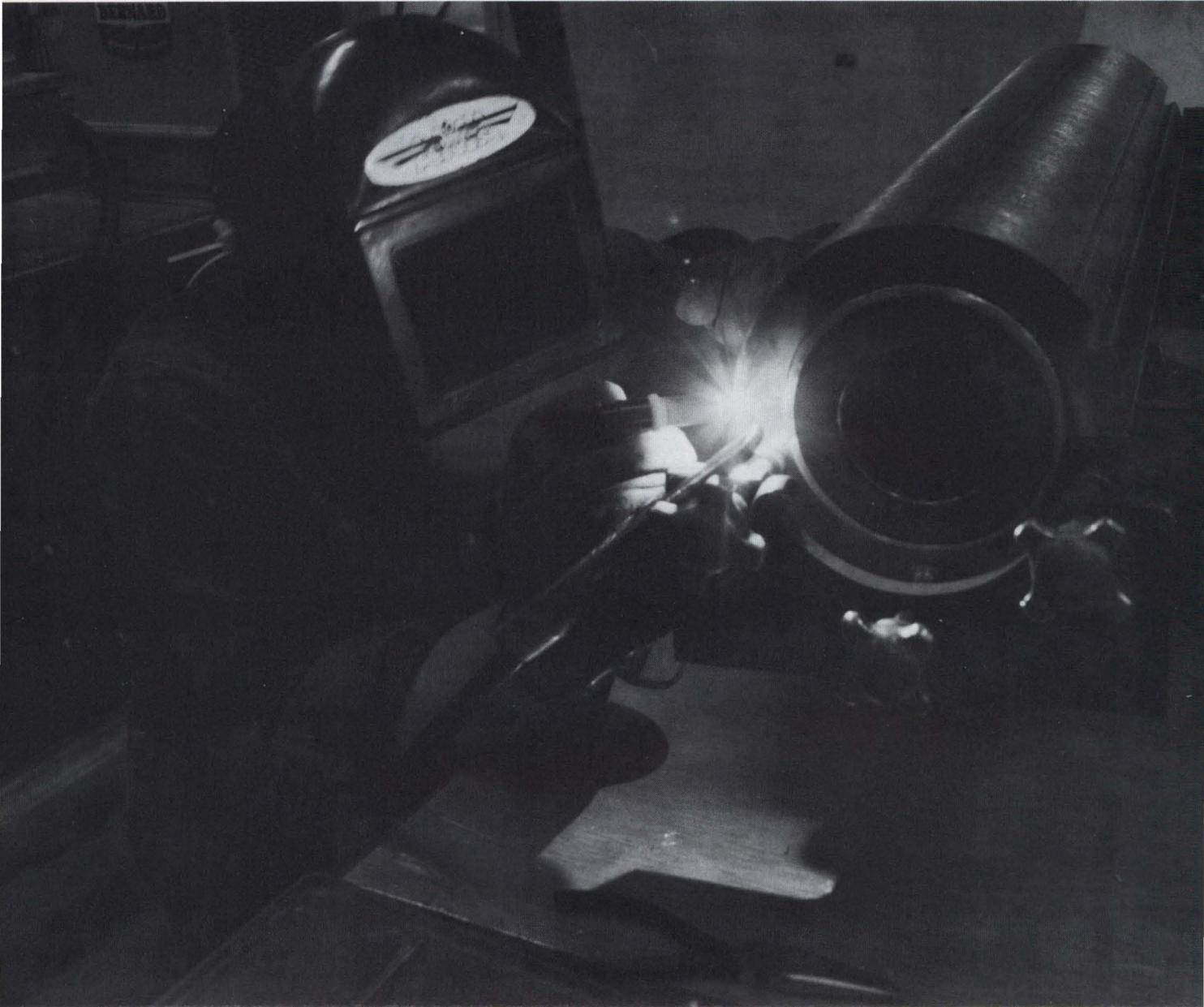
A welder at work on a correction coil being built by Research Services for the Energy Saver.
