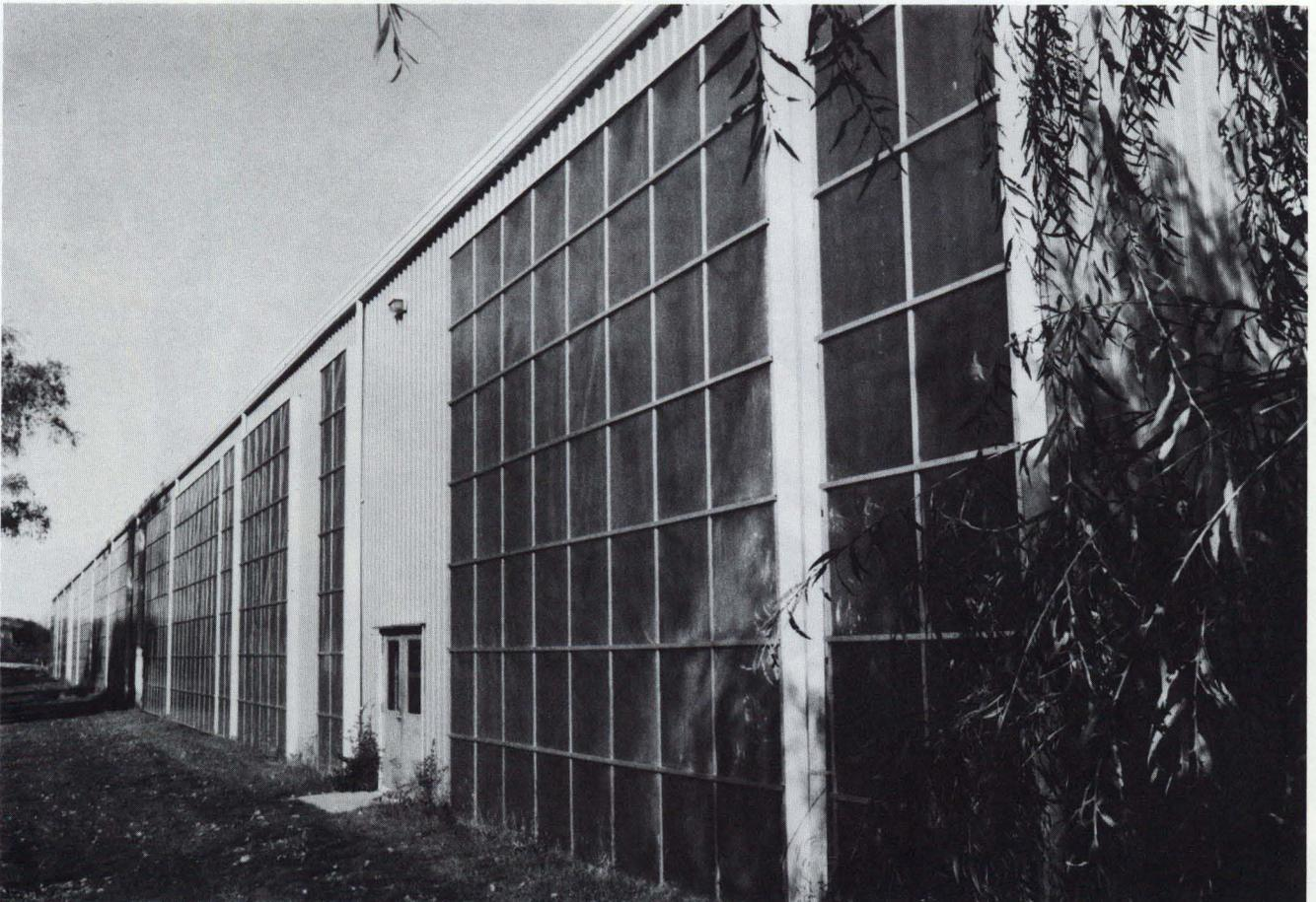
Passive solar wall on the warehouse.
