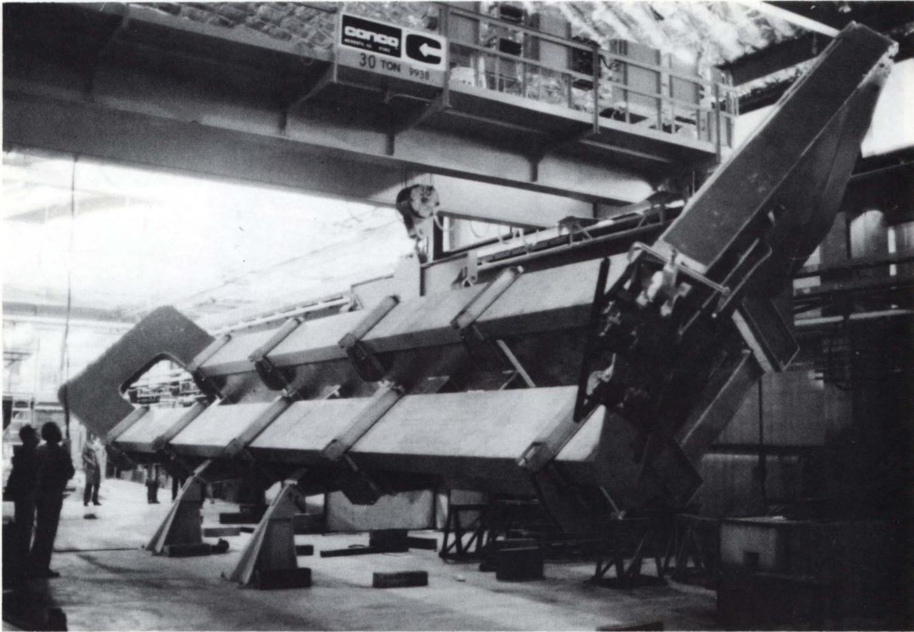
Four-layer coil tipped on its side for installation in the magnet yoke in the Meson Detector Building.
