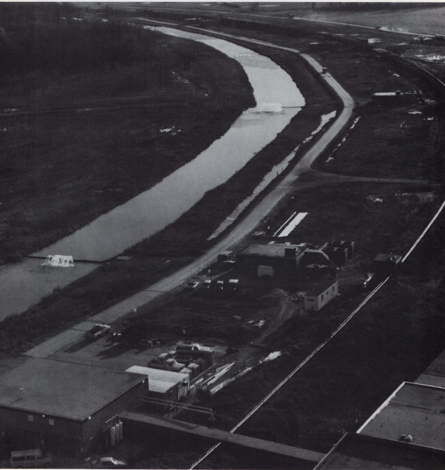
A view from Wilson Hall with the helium transfer line on top of the Main-Ring shielding berm. The Transfer Hall is at the lower right, the A0 assembly area and the F4 service building are at the left. The other F service buildings and the RF Building march off into the distance.
