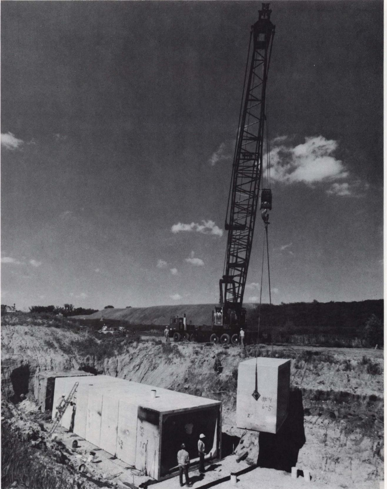
A concrete tunnel section for the Enclosure H extension being installed.
