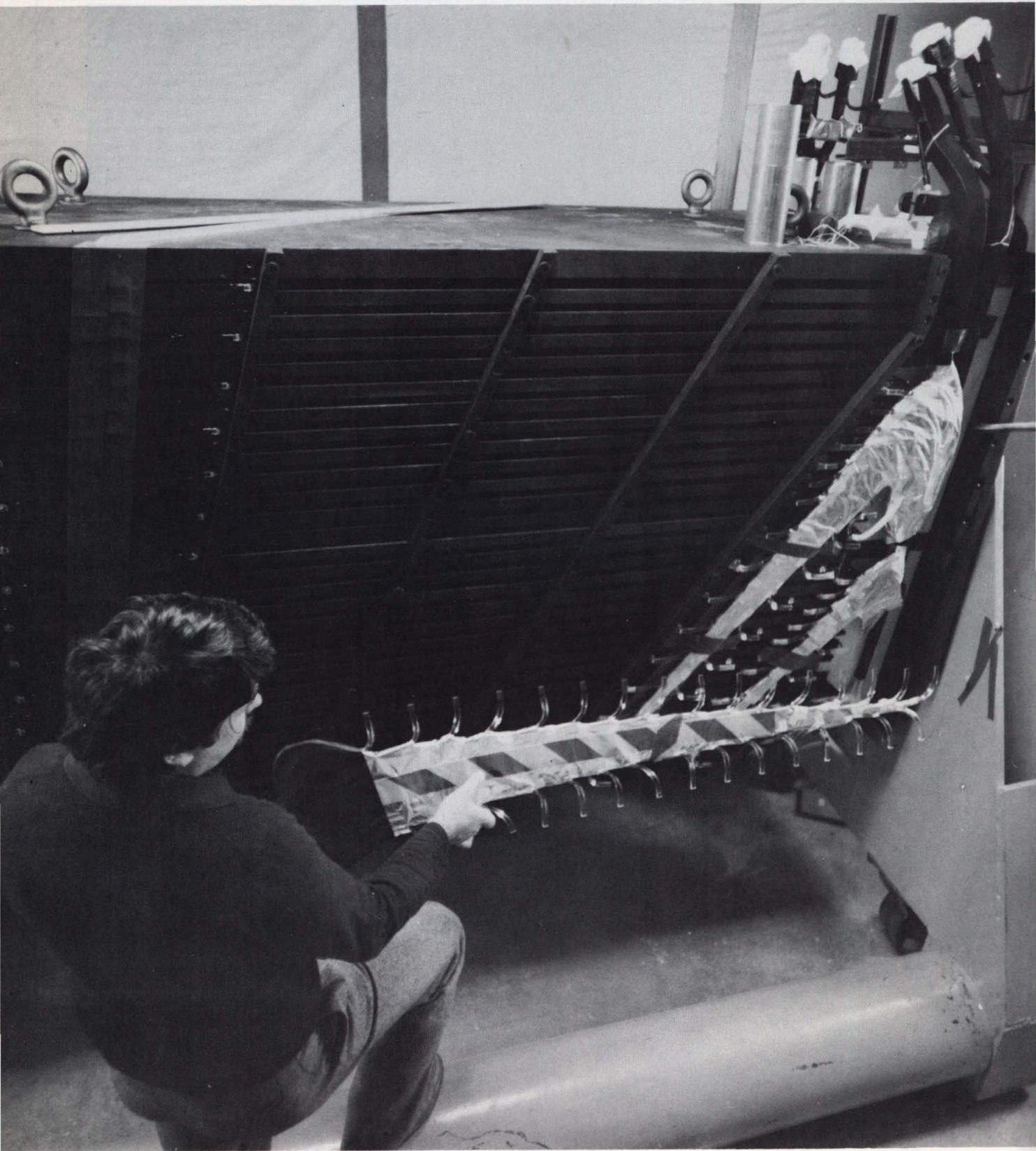
Sergio Bertolucci of Frascati checks a model of a central calorimeter for the Collider Detector.
