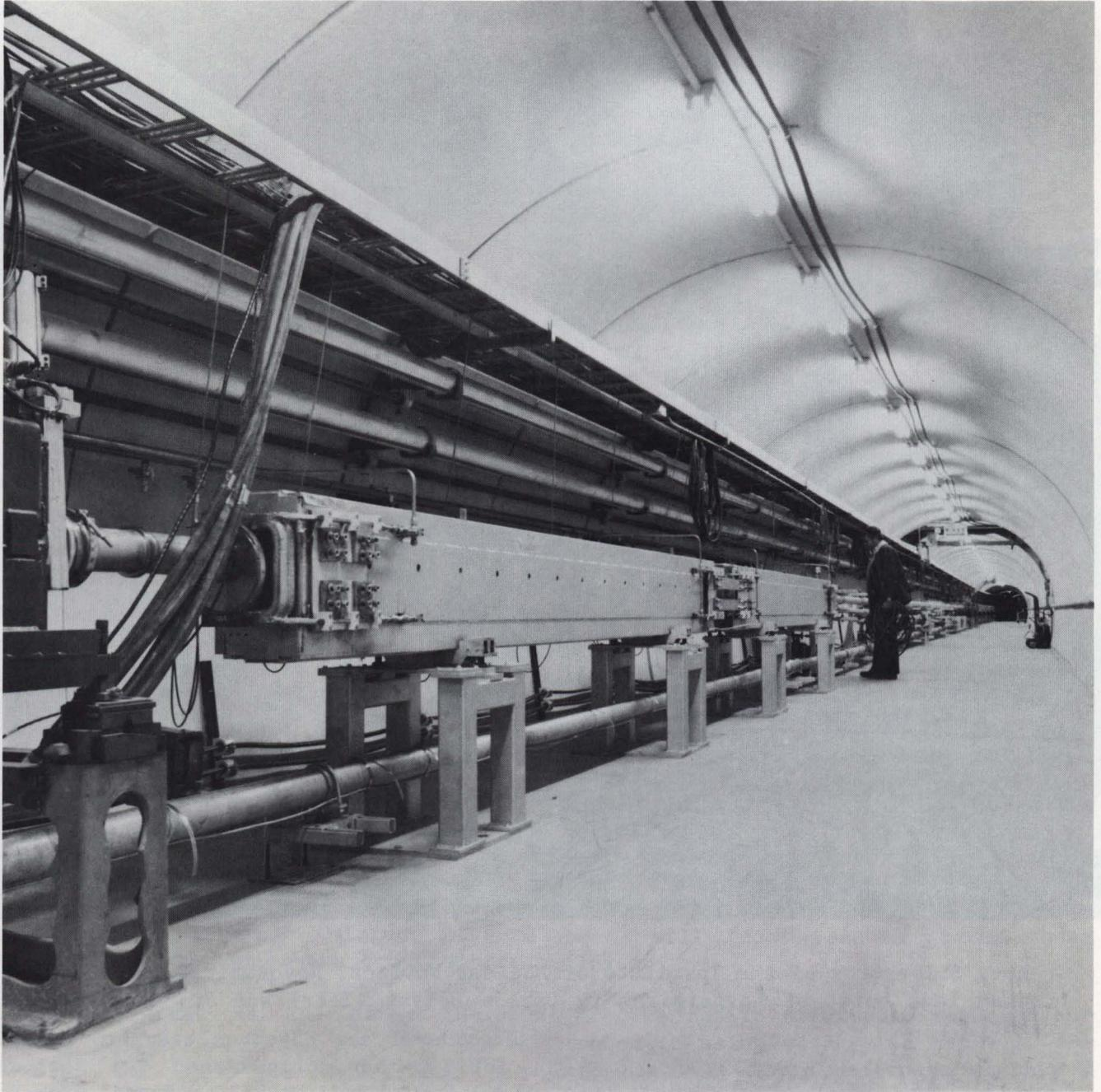
Leon Bartelson at the Saver injection line in the E0 straight section where 150-GeV beam will be bent downward from the Main Ring above to the Energy Saver below.
