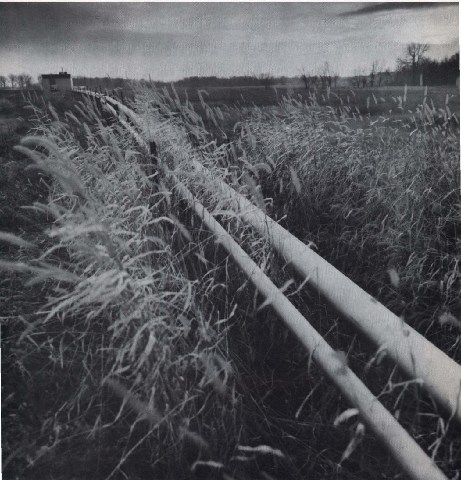
A closeup view of the helium transfer line on top of the berm.
