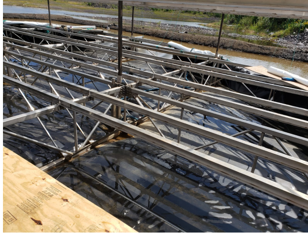
Figure 5: Rows of stringers bolted onto the main support structure. Instrumentation would be attached onto the top of the stringers.
