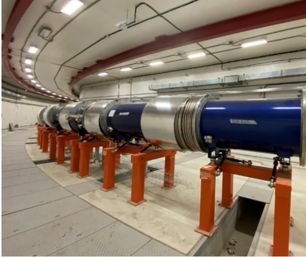
Figure 9: Assembling of Collider arc magnets.
