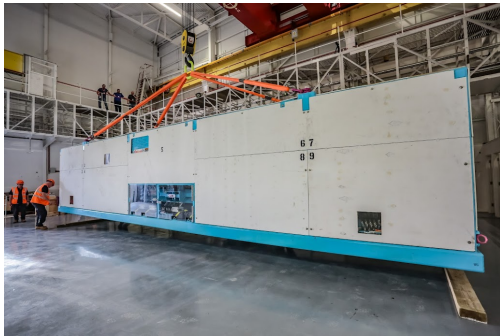
Figure 5: Transport System during unloading at STFC-UKRI with bespoke bale and slings.
