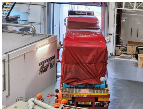
Figure 9: Trailer after delivery at STFC-UKRI. Note sharp trailer angle relative to the entry door to avoid the experimental hutch (left).
