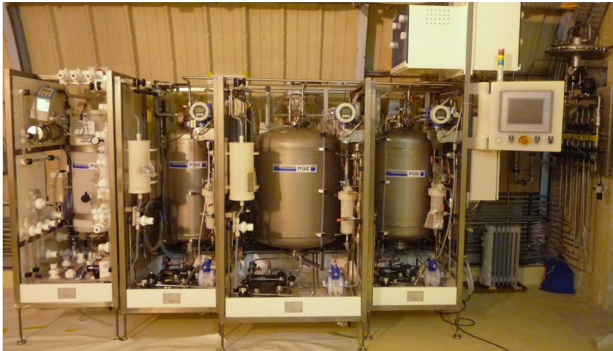
Figure 9: Detector Fluid Operating System installed in the underground laboratory of the far detector. From left to right are shown: Target, GC, buffer and veto liquid systems; the control unit including gas touch screen; the over-, underpressure safety and low pressure nitrogen boxes, and one of the gas system manifolds.
