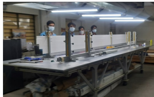
Fig. 4 Assembly of di-counter wall in progress.
