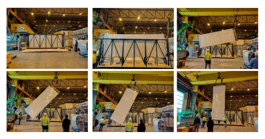
**Figure 70**: Arrival of an APA in EHN1 and its positioning. The upper left image shows the orientation of the APA as delivered, the lower right shows its vertical orientation when it is lowered into the material sas.
