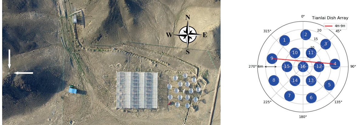
Figure 1. Left: Top view of the Tianlai Dish Array Pathfinder and Cylinder Array Pathfinder taken with a DJI M600 Pro drone at a height of 280 m above the ground. The position of the calibration CNS is indicated by the white arrows on the left. The relative distance vector from the feed in dish 16 at the center of the array (when pointed toward the zenith) to the CNS is [-184.656, 13.915, 12.588] meters, with x,y,z to the east, north, and zenith. Right: A schematic diagram of the Tianlai Dish Array; 0^\circ coincides with North. The dishes are arranged in two concentric circles of radius 8.8 m and 17.6 m around a central dish. The dishes have dual-linear polarization feed antennas with one axis oriented parallel to the altitude axis (horizontal, H, parallel to the ground)) and the other orthogonal to that axis (vertical, V). For example, shown in red is one of the baselines that is studied later in this paper, the H polarization of dish 4 correlated with the H polarization of dish 9: 4H-9H. Other baselines used later in the paper use the same naming convention.
