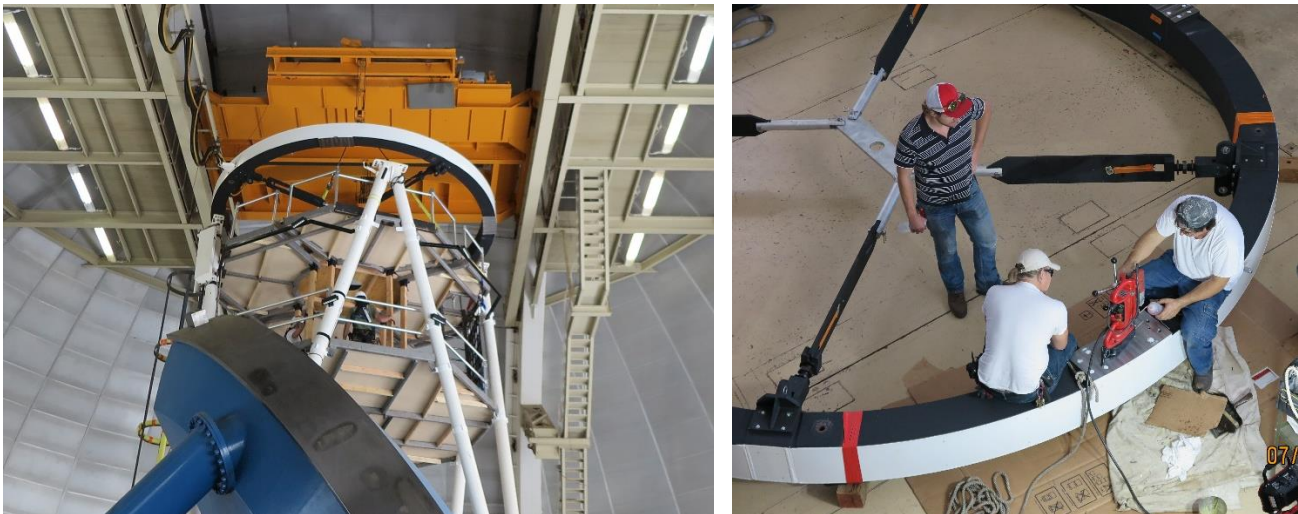
Figure 3: Left-The pre-tensioned DESI upper ring being lowered by the 5-ton dome crane onto the top of the Serrurier truss for alignment, match-drilling, and transferring the locations where holes are to be tapped into the ring for its mounting bolts. The four pairs of struts comprising the Serrurier truss are held in place by the two-level, temporary work platforms, which were installed prior to removal of the old upper assembly. Right-NOIRLab personnel field-tapping the bottom side of the DESI upper ring at the locations marked during the operation shown in the left photo. The pre-tensioning system, consisting of the four DESI middle vanes and a custom spreader assembly in the center, remains in place and tensioned, to allow test-fitting of the ring and fasteners to the Serrurier truss.
