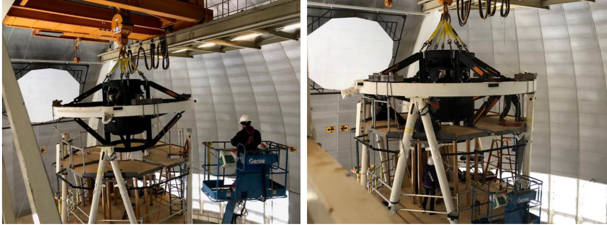
Figure 9: Left-The DESI upper assembly is lowered onto the Mayall Serrurier truss. Right-Kitt Peak personnel finalize the fastening of the ring with the truss.
