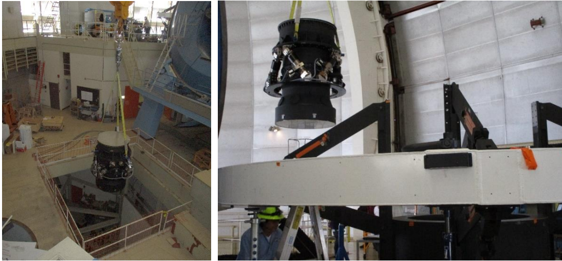
Figure 7: Left-The DESI corrector and hexapod being lifted from the ground floor through the open hatch in the M floor, just north of the blue telescope mount. The ring and vane assembly is visible near the top right of the photo on the C floor,
