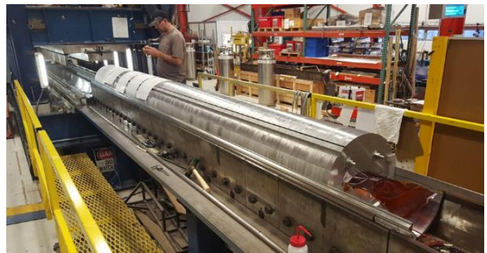
Fig. b5. Upper yoke sections being installed
