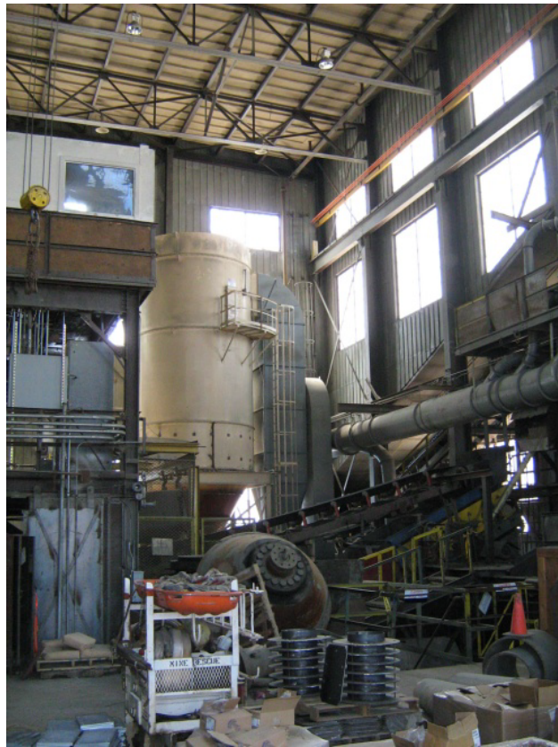
Figure A-24: Photo of Yates Crusher interior. (HDR)
