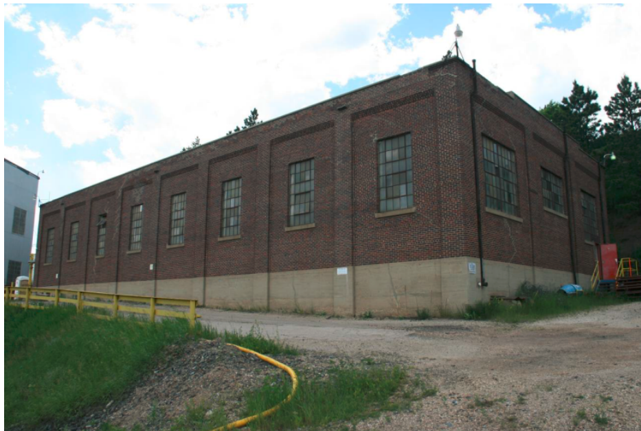
Figure A-20: Photo of Ross Dry exterior. (HDR)
