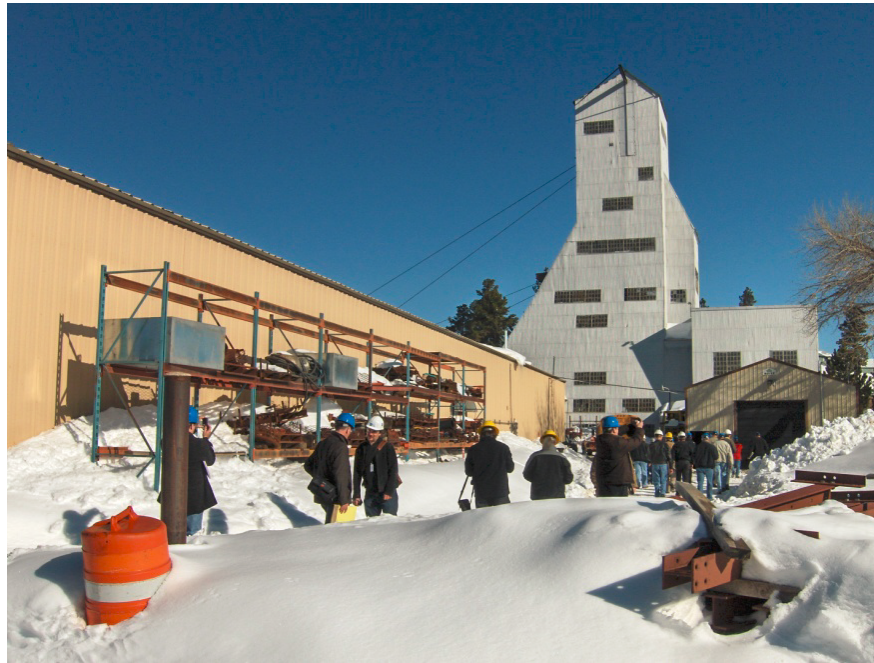
Figure A-18: Photo of Ross Headframe. (HDR)
