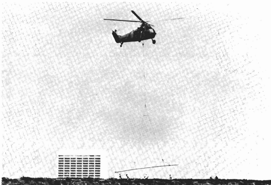
Fig. 5. Installation of eighty foot section of transfer line for the Doubler with a helicopter.
