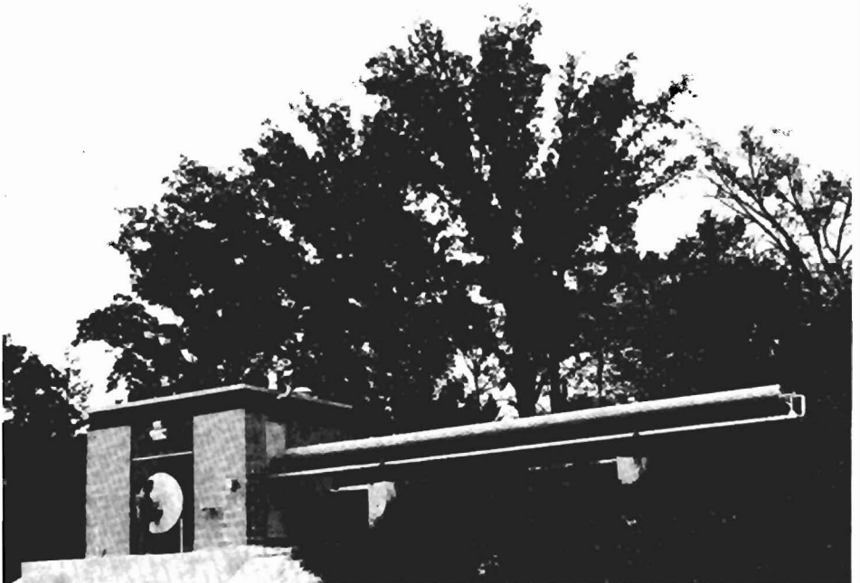
Fig. 7. Refrigeration building with horizontal exchanger column.
