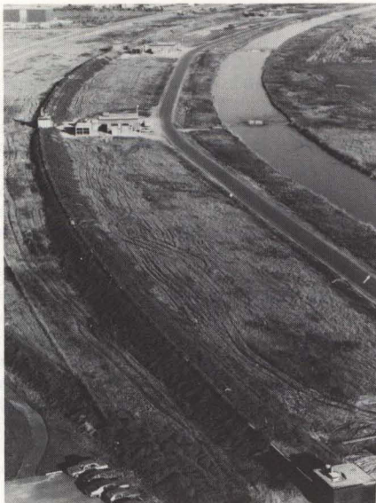
Fig. 1. View of Fermilab tunnel from Wilson Hall. Note the Central Helium Liquefier at the upper left as well as the satellite refrigerator buildings and the helium transfer line on the berm.
