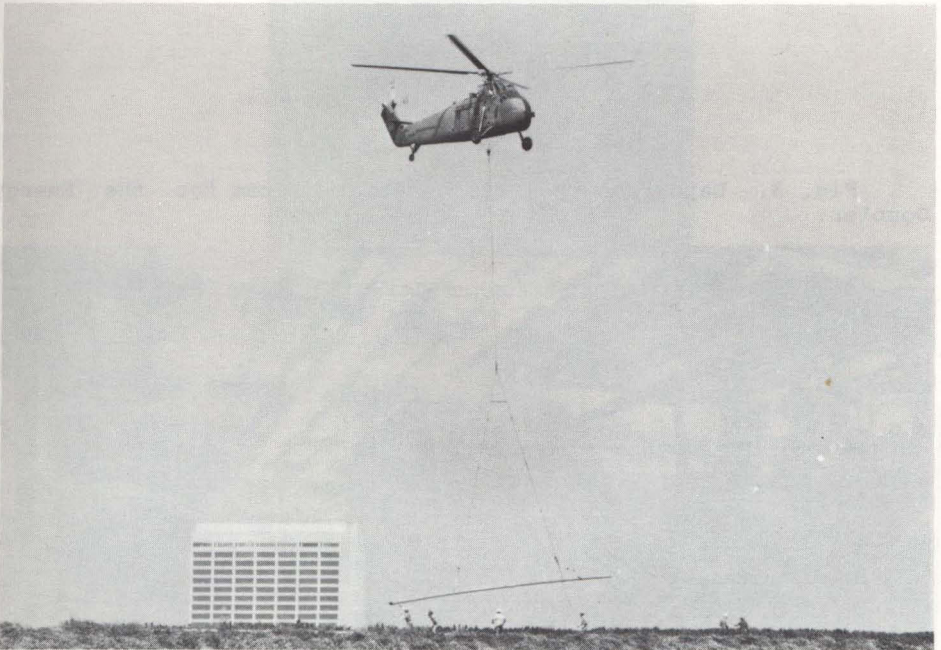
Fig. 5. Installation of eighty foot section of transfer line for the Doubler with a helicopter.
