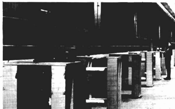
Fig. 5. Laser and target monuments used on the 805 MHz linac support structure.
