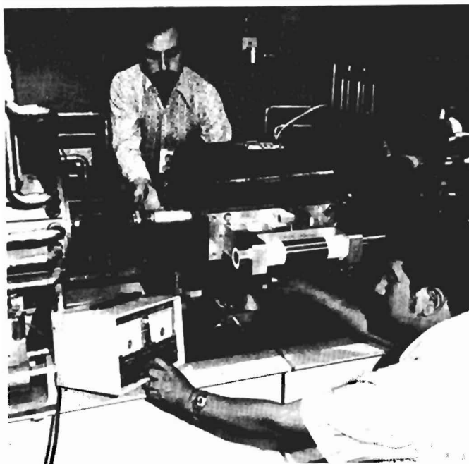
Fig. 16. Installation of quadrupole doublet between 805 MHz linac modules. Laser fixture is shown on doublet.
