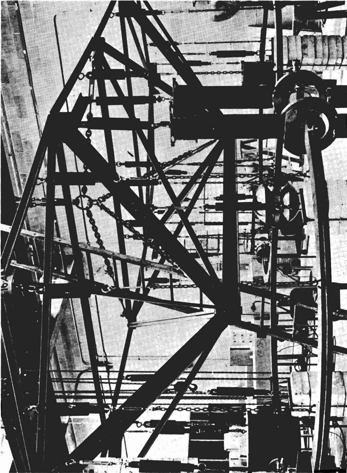
Fig 5 - Vacuum chamber suspended by the steel spider
