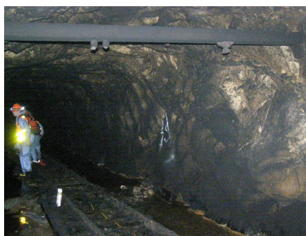
Figure 2. Station 308 in the Pioneer Tunnel during recent reconnaissance [5].
