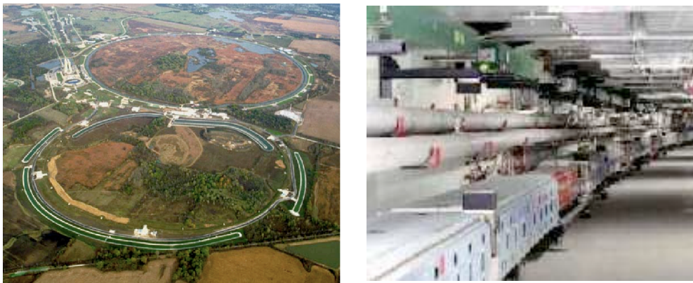
Figure 4.5: Left: Aerial view of the Main Injector (front) and the Tevatron (back). Right: Main Injector Tunnel. The lower magnets are part of the Main Injector, the upper green magnets are part of the Recycler.
