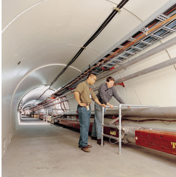
Figure 2.5. The Tevatron was built in a tunnel that used to hold another accelerator above it. As the Tevatron began operation, the Main Ring accelerator was removed. The Tevatron magnet in the photo above is painted red.
