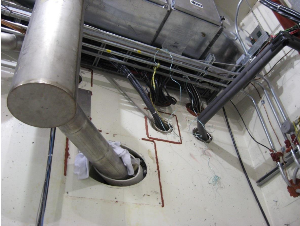
Figure 1. Large (up to 10”) penetrations near ceiling of MTA experimental hall for cryogenics.
