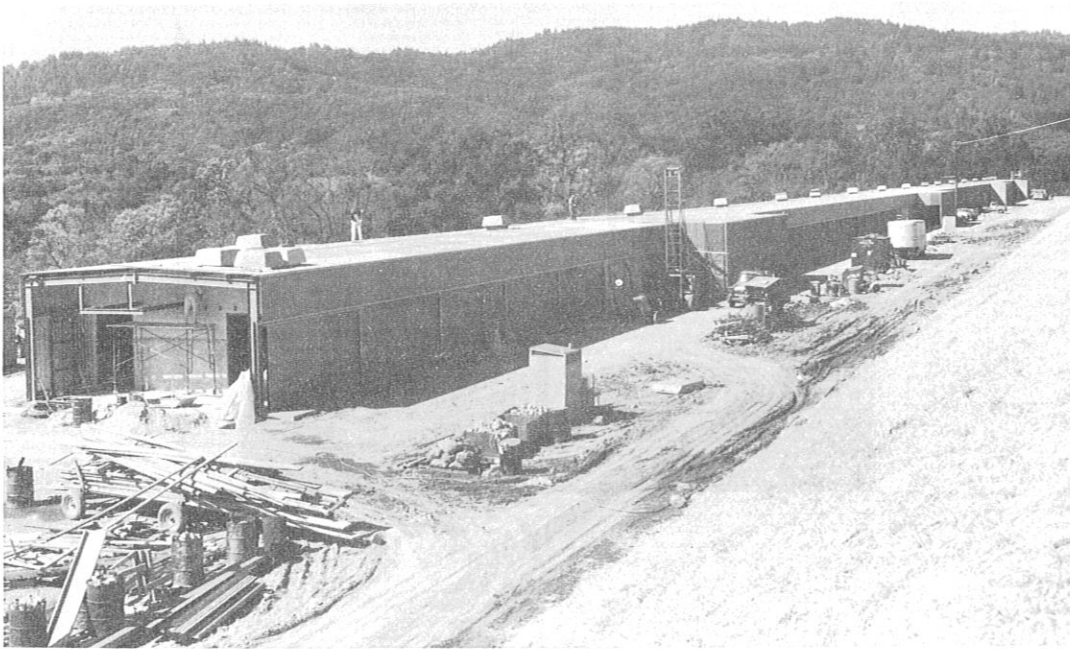
Fig. 4 Beginning of klystron gallery construction.
