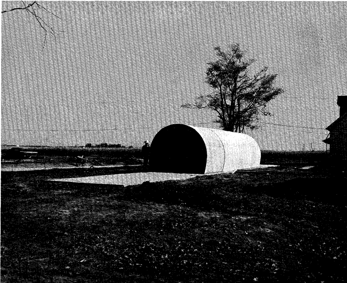
Fig. 3. Precast Main-Ring tunnel sections. Vernon Kenney of AEC is to the left.
