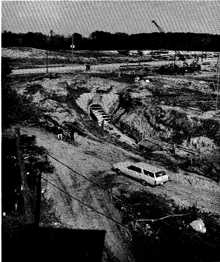
Fig. 1. Work on the last part of the Booster tunnel.
