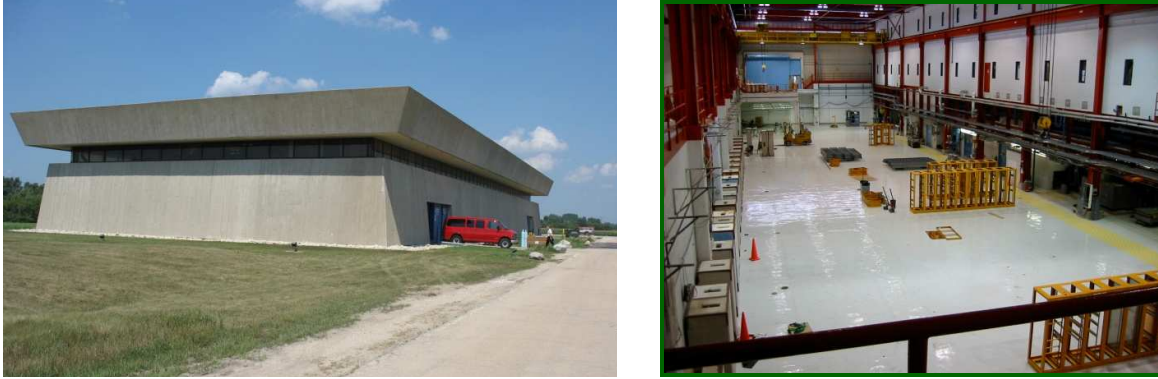
Figure 4.1: a) The New Muon Lab building; b) the ILC Test Facility at the New Muon Lab.
