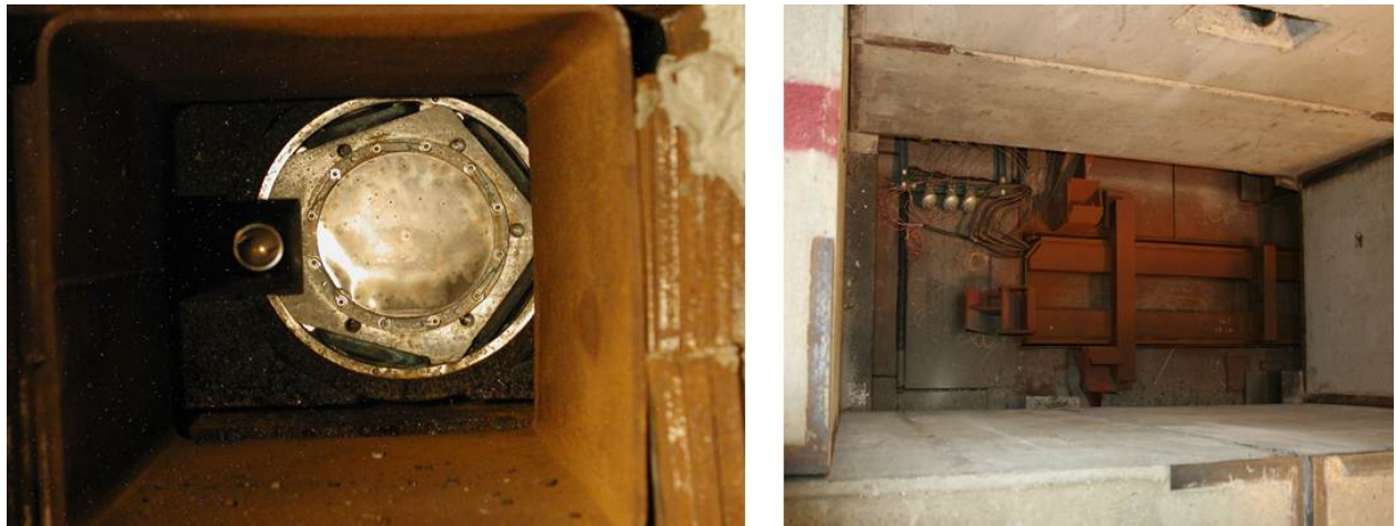
Figure 7.24: ( left ) Photo of the front face of the beam dump as taken in 2003. ( right ) Looking down on the top of the dump plug below the surface of the shielding blocks .
