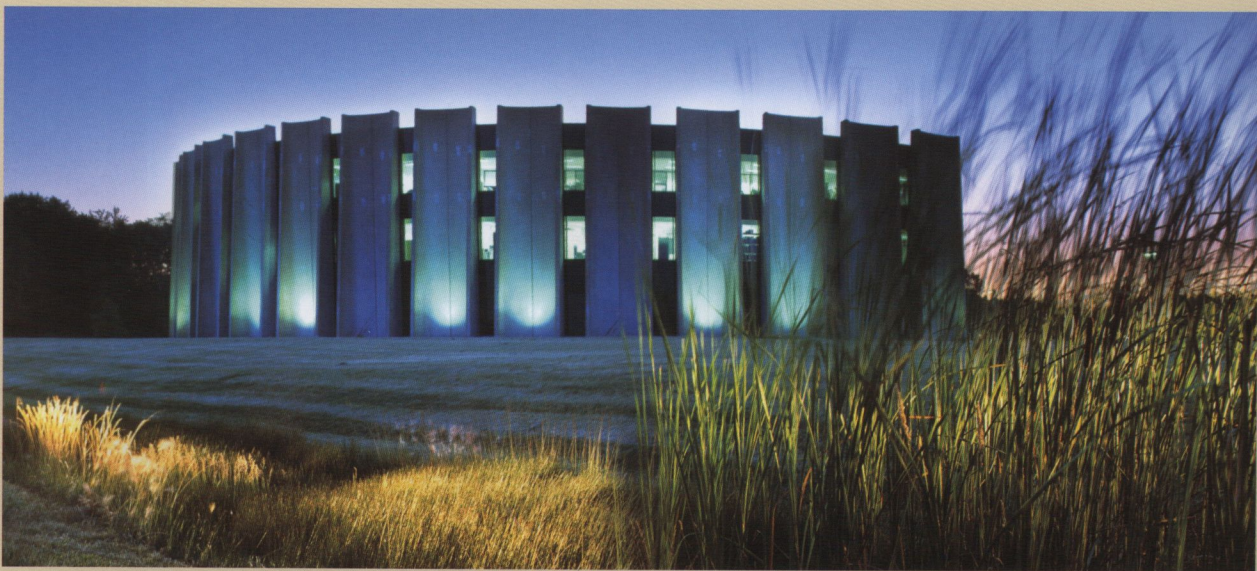
The Feynman Computing Center, is a three-story semicircular structure of 74,000 square feet which houses the central computing facilities for the Laboratory. The building's pre-cast concrete backbones are supported on a steel frame, as is the north-facing glass facade. The pre-cast panels provide protection from the sun's heat and also duplicate the vertical lines of Ramsey Auditorium to the south. (Photo credit Peter Ginter).
