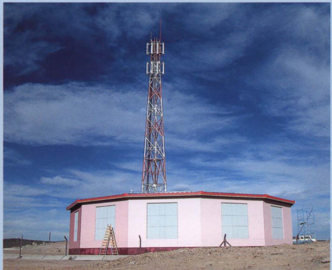
The recently finished third (of four) fluorescence detector buildings at the southern hemisphere Auger site in the Province of Mendoza, Argentina. Behind the detector building is a communications mast that transmits data from the fluorescence and surface detectors to the data acquisition center on the Central Campus.
