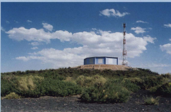
Los Leones is the first of 4 fluorescence detector buildings at the southern hemisphere Auger site in the Province of Mendoza, Argentina. The communications mast collects data from surface detectors, as well as fluorescence detector data from Los Leones, for relay to the data acquisition center on the Auger campus.
