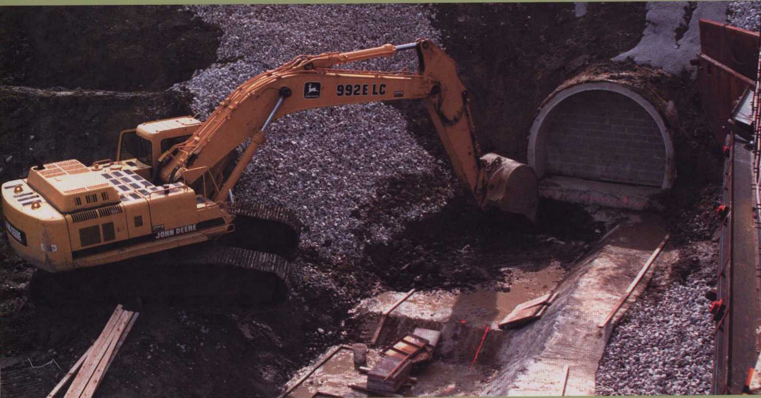
Civil construction for the Main Injector project
