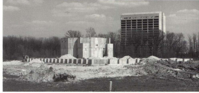
(Above) A science laboratory with stations for 40 students, a classroom and office space are included in the Science Education Center.
