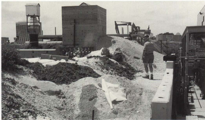
On the berm to the south of CDF, John Grimson checks out the earth coverage over the pieces of iron designed to give additional shielding in the B0 region.
