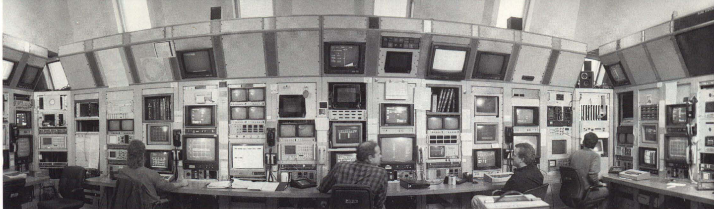
In the Main Control Room, Fermilab personnel use an array of computer screens to monitor parameters — such as beam current, position, and vacuum — to insure the smooth and efficient operation of the accelerator around the clock.
