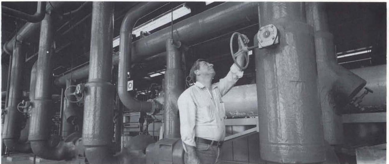
*Fred Randazzo adjusts the water flow from the chilled water system in the Central Utility Building. The chilled water circulates through heat exchangers to cool the low conductivity water crucial for cooling the conventional magnets in the Booster and Main Ring. The chilled water also goes to air conditioning coils for Wilson Hall.*
