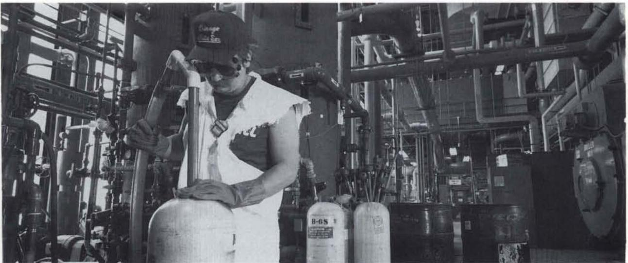
*Walter Canning empties resins from deionized water tanks into the main regenerating tank at the Central Utility Building. This regeneration procedure is a routine function that maintains the high purity level in the chilled water systems.*
