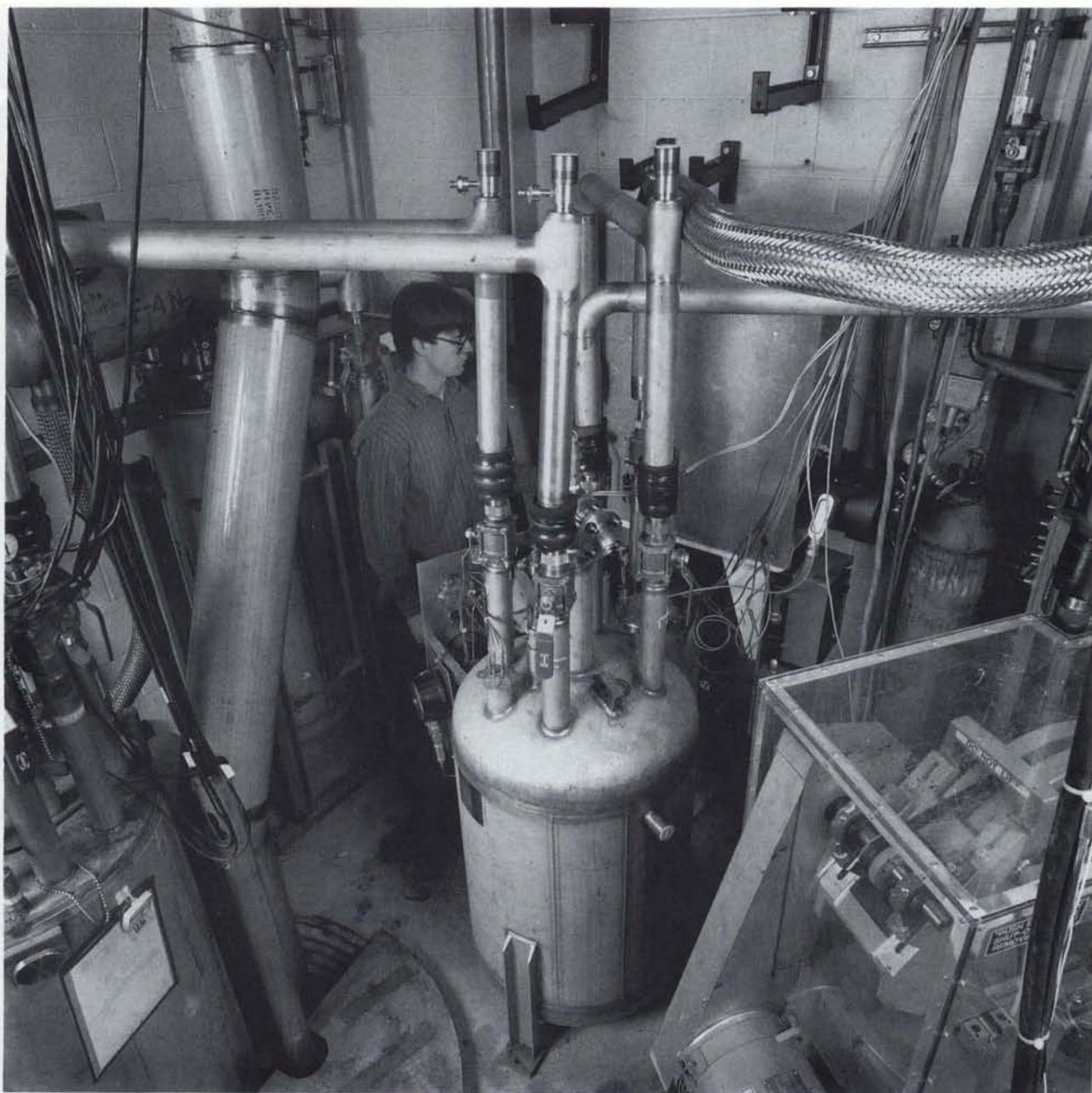
*Joel Fuerst of the Accelerator Division cryogenics group monitors the operation of a cold helium compressor in a satellite refrigerator.*
