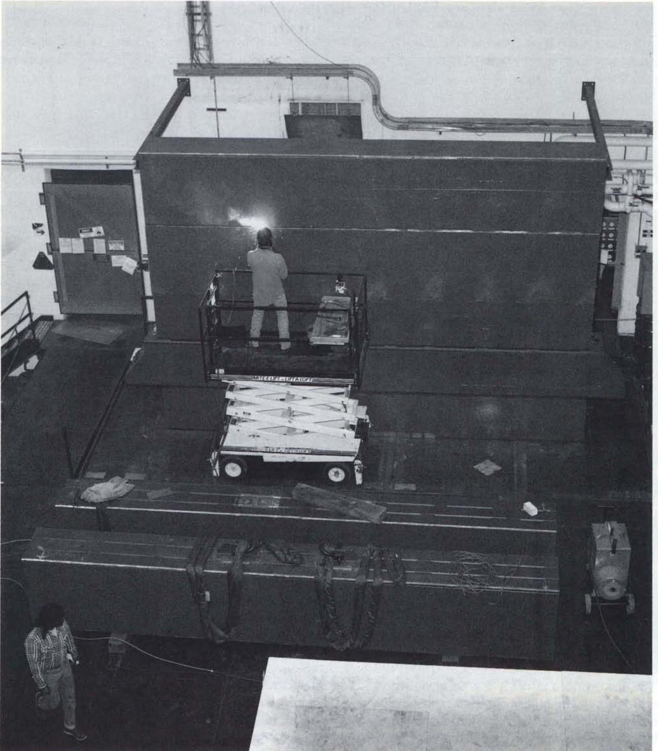
*Construction of a new steel absorber wall for CDF will allow the detector to more cleanly identify penetrating muons emitted in proton-antiproton collisions.*
