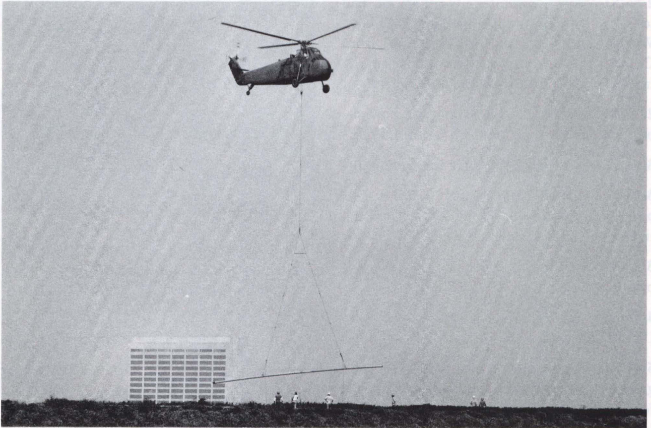
Helicopter-aided installation of the Helium Transfer Line atop the Main Ring berm, July 10, 1981.
