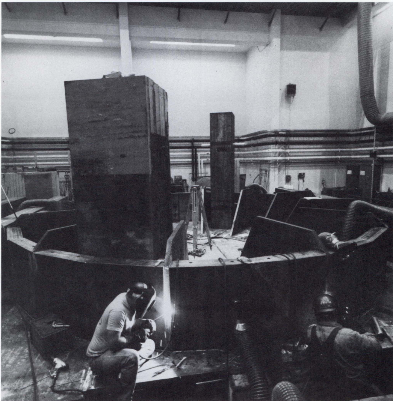
Welding the support ribs on the magnet end wall.
