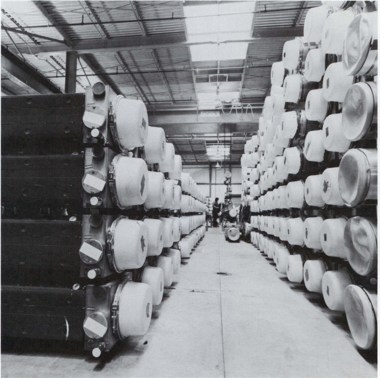
Completed, accepted Energy Saver magnets in Industrial Building 4 awaiting tunnel installation.
