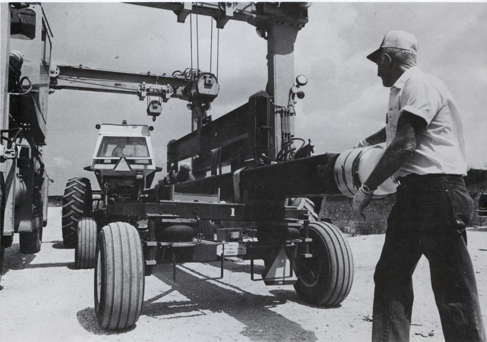
Harry Krider, a Belding employee, unloads Energy Saver magnets at D0 prior to being lowered into the tunnel for installation.
