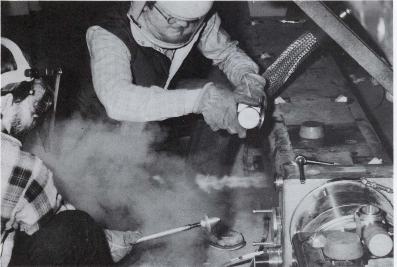
Ken Olesen (left) readies a temporary blankoff plunger while Jay Theilacker removes a malfunctioning liquid helium relief valve from an Energy Saver dipole magnet.
