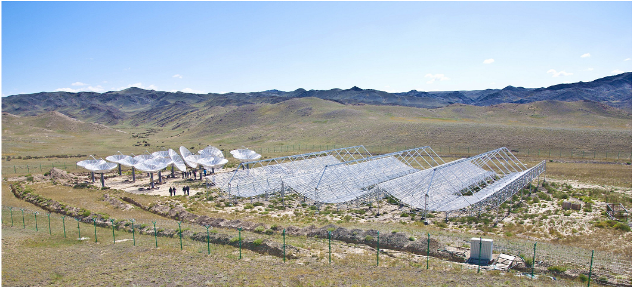
Figure 2. The photograph shows the Tianlai Pathfinder dish and cylinder arrays. The dish array is an array of 16, fully-steerable, on-axis dish antennas, each 6 m in diameter. A dual-linear polarization feed is located at the focus of each dish. The cylinder array consists of 3, fixed, cylindrical reflectors, each 15 m wide and 40 m long, placed side-by-side (in the E-W direction) with their long axes oriented along the N-S direction. A linear array of dual-linear polarization feeds is arranged along their focal lines. The photograph is taken looking toward the southeast.
