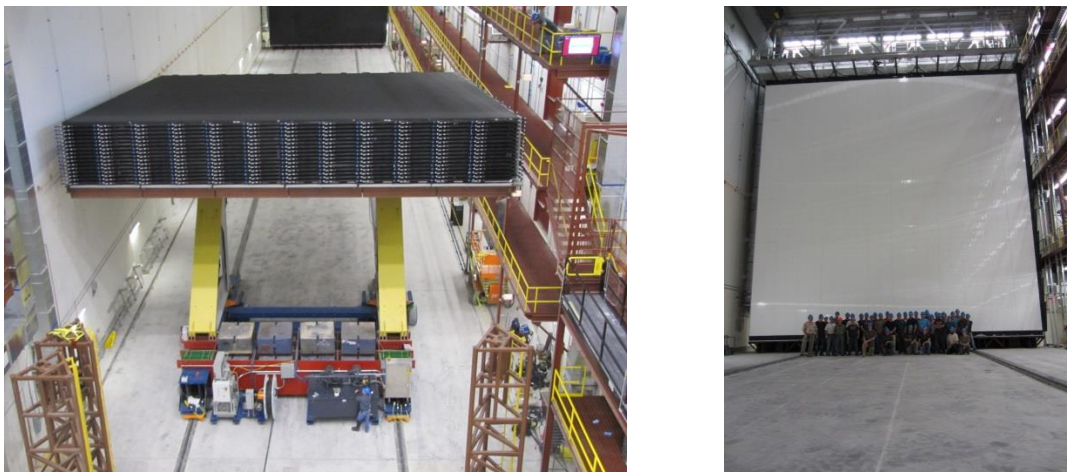
128 129 Figure 4: (a) One of 28 Far Detector Blocks is moved into position with the Block Pivoter. (b) A Block is in its final position. The 130 installation crew of 38 people sets the scale perspective. The outside surfaces of Blocks are painted black to prevent external light 131 from passing through the PVC material and being sensed by the APDs.
